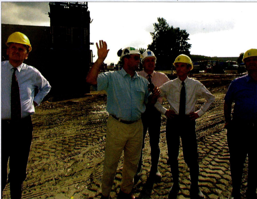
Chief scientific adviser to the UK Government, Sir Robert May (second from right), inspects construction work for CERN's LHC project with (left to right) UK CERN delegate Ian Halliday , CERN engineer Tim Watson , LHC project director Lyn Evans and CERN Scientific Policy Committee chairman George Kalmus .
